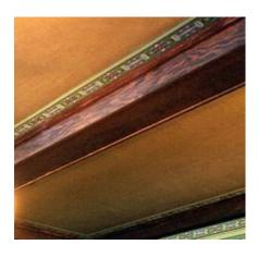
**Sheetrock** - This is normal sheetrock or wallboard painted with enamel, latex or flat paint. The enamel and latex paints allow the spray/wipe technique to be used. Flat paint ceilings should be repainted when they become soiled since the flat paint can be removed with mild agitation or detergents.
